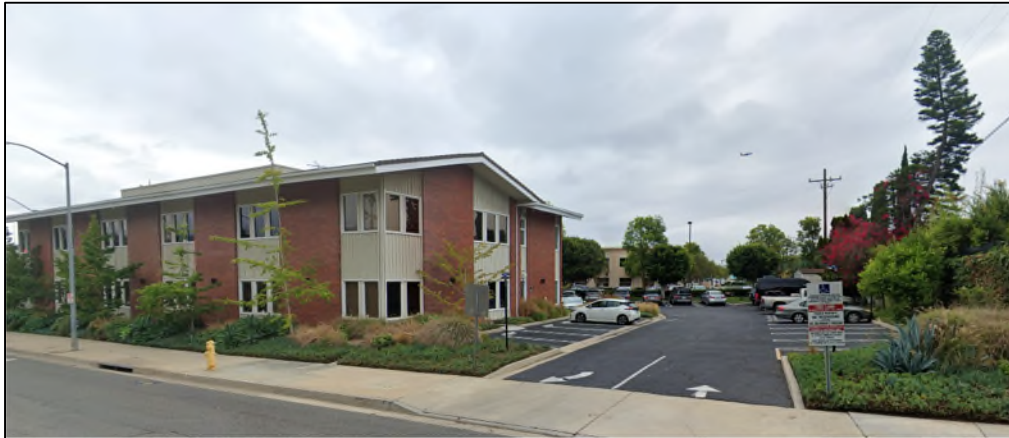
View from Newport Boulevard
