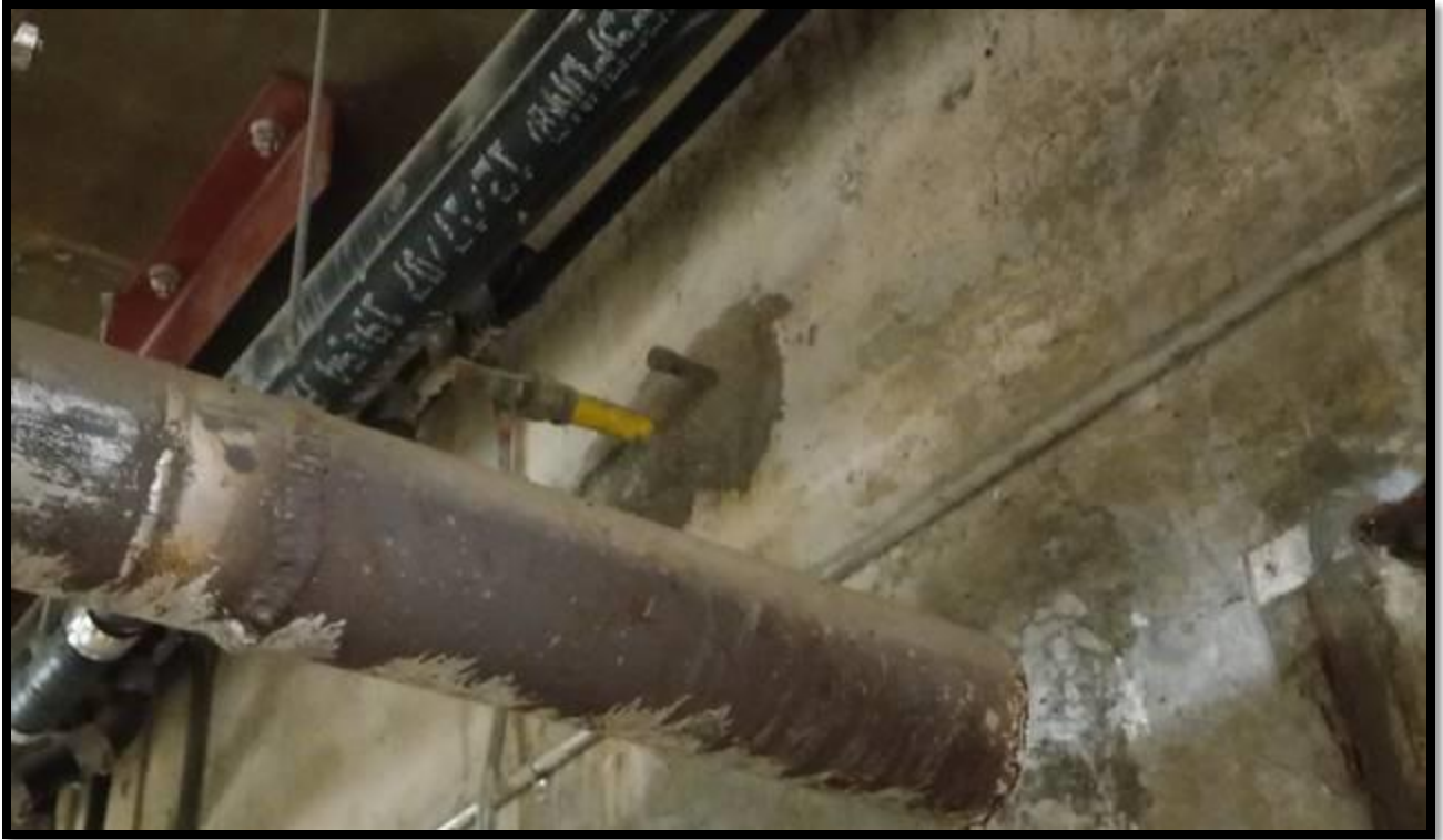
Figure A1.2.1 – Existing pipes from the tank have been capped and the holes patched inside the basement wall.
