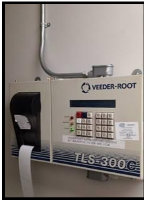
Figure A1.1.1 - As part of the base bid Contractor shall disconnect and remove the Veeder Root Box in the Police Department basement. Existing low power shall be capped in a covered electrical box.
